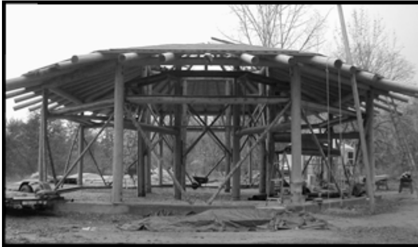
Common House roof decking nears completion - November, 2004
